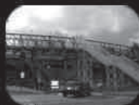
Bridge Construction Update
